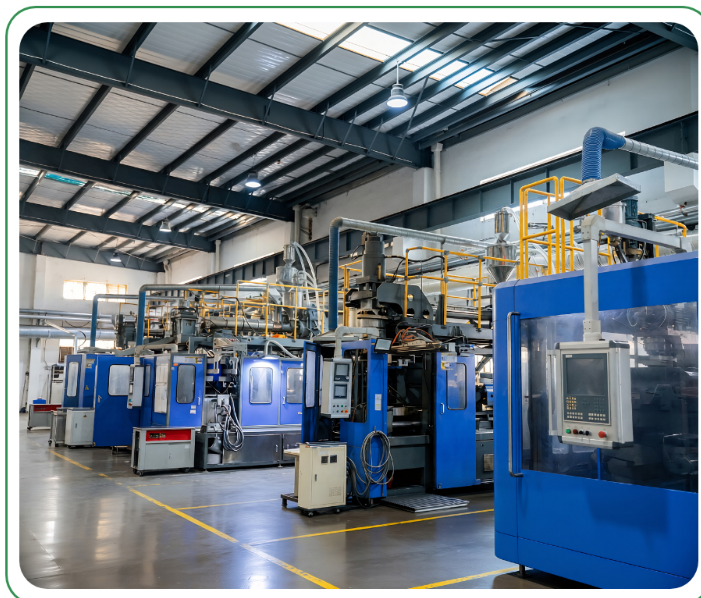
吹塑生产线 Blow Molding Lines
